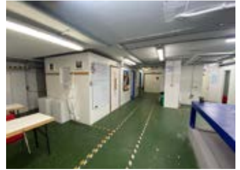
The basement 'before'
